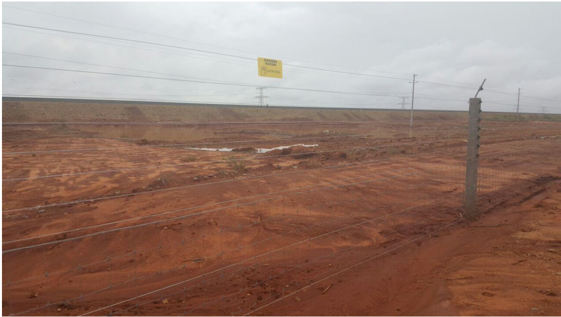
Plate 5: a) Elephant-proof electric fence as designed by KWS and submitted to the SGR constructors, and b) a 200 m section of trial elephant-proof fence under construction around Manyani shopping center as at November 2016.
