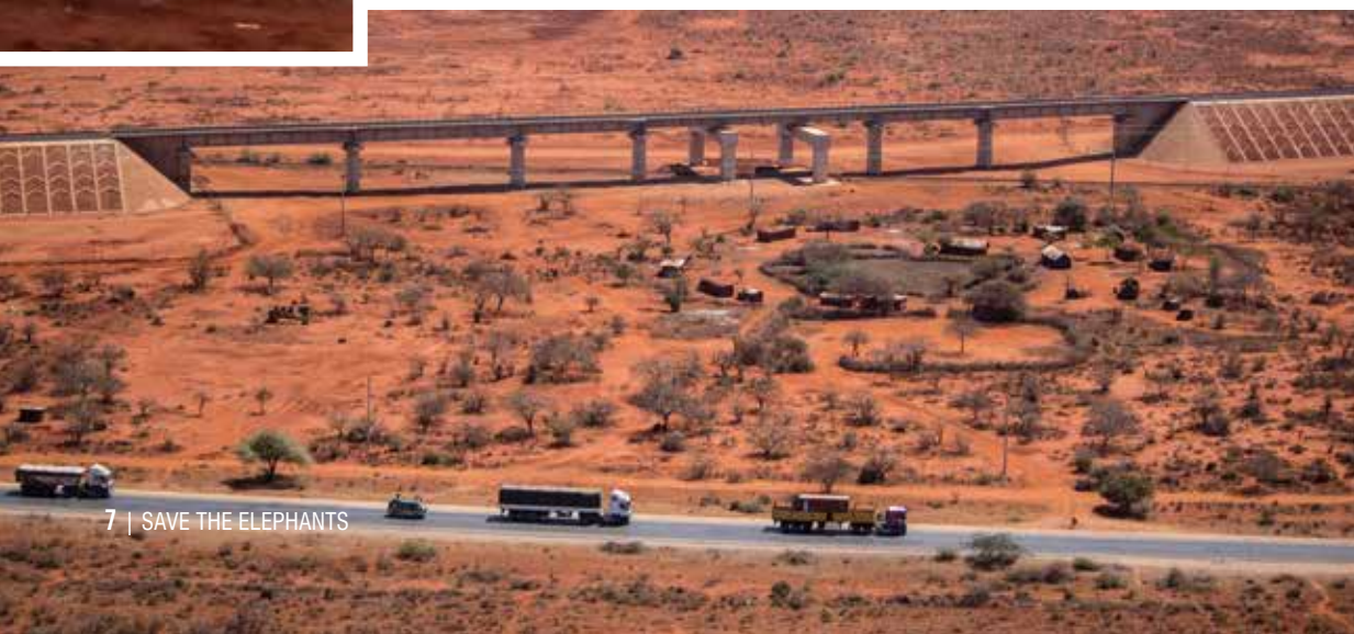
Below: Underpasses beneath the fast rail link between Nairobi and Mombasa were built to allow wildlife movements through the Tsavo Conservation Area to continue. For them to work they must be kept free from settlement, unlike this one pictured, and align with crossing points across other infrastructure like roads.
